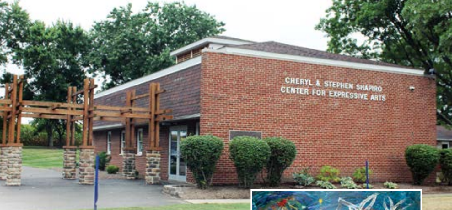
Above: The Cheryl and Stephen Shapiro Center for the Expressive Arts on the Wooster Campus of The Village Network.
